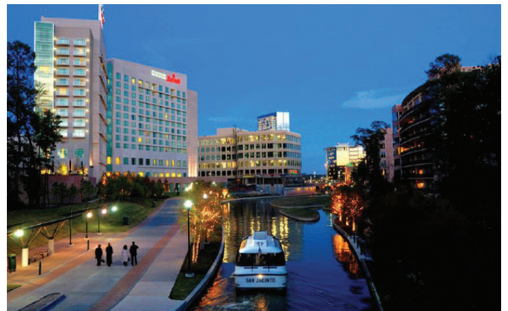
THE WOODLANDS, TEXAS. The Woodlands project, one of the largest hotel mixed-use developments in the United States, demonstrates how each component of a hotel mixed-use project enhances the other. Residential elements fetch higher prices and rents, retail and restaurants generate more sales, and hotels achieve significantly higher revenue per available room (RevPAR).
