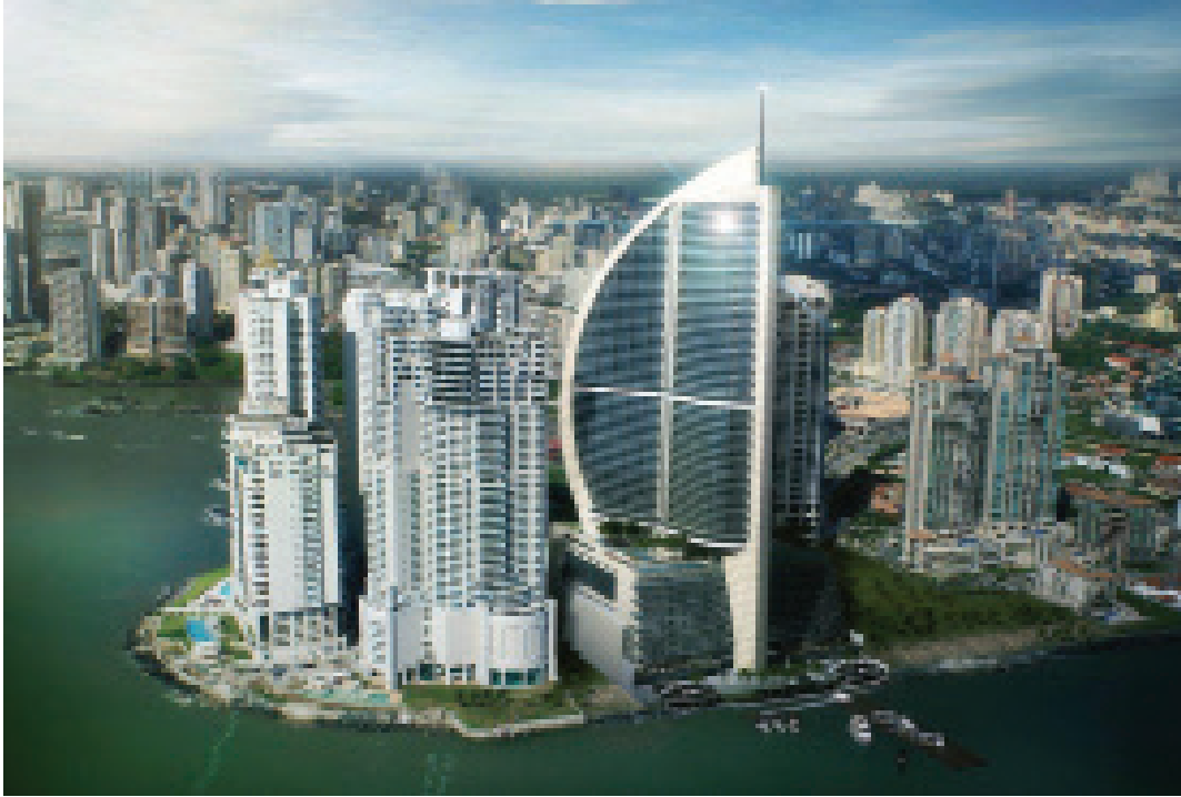
TRUMP OCEAN CLUB INTERNATIONAL HOTEL & TOWER, PANAMA CITY. Luxury hotels like this often provide the spark plug to energize and create value with high-end mixed-use for hotel-anchored residential, condo hotel, retail and office projects. We have represented the Trump Organization and other clients on more than 100 hotel mixed-use projects throughout the U.S., Latin America, the Caribbean, Asia and Europe.
