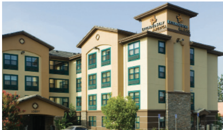
EXTENDED STAY AMERICA, SACRAMENTO. We have performed system-wide accessibility audits for Extended Stay America hotels (including prototype plan checking), and have assisted them nationally with proactive and defensive ADA and related accessibility compliance matters.
