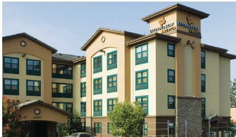
EXTENDED STAY AMERICA, SACRAMENTO. We have performed system-wide accessibility audits for Extended Stay America hotels (including prototype plan checking), and have assisted them nationally with proactive and defensive ADA and related accessibility compliance matters.
